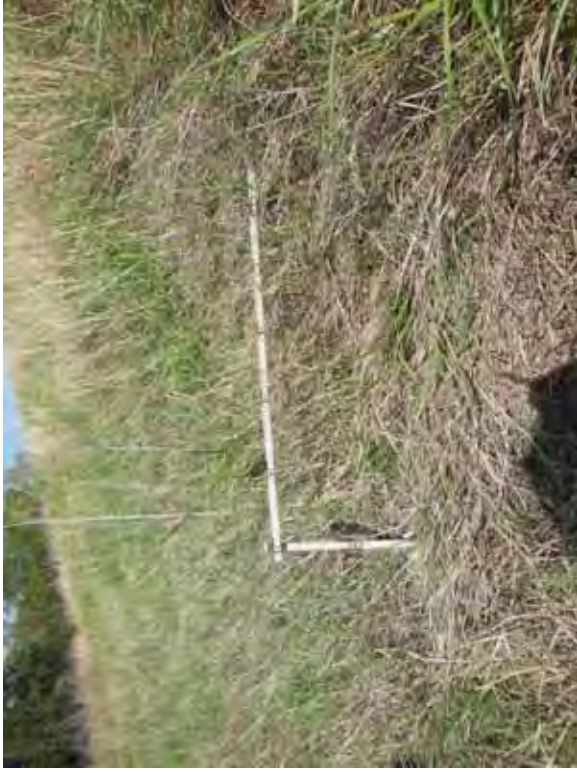
Photo 86: South embankment exterior slope measured approximately 3H:1V.
