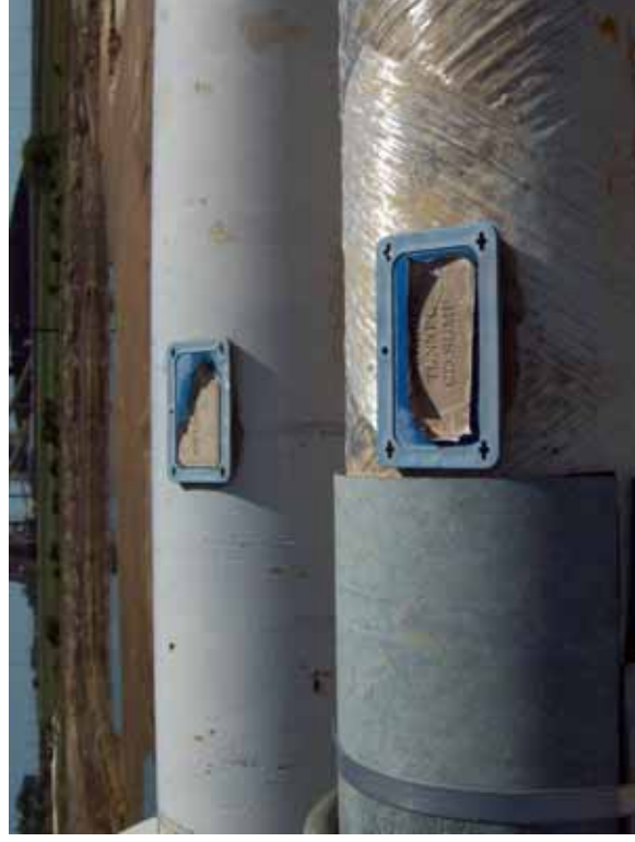
Photo 36: Labels for left two 6-inch-diameter inlets shown in Photo 34.
