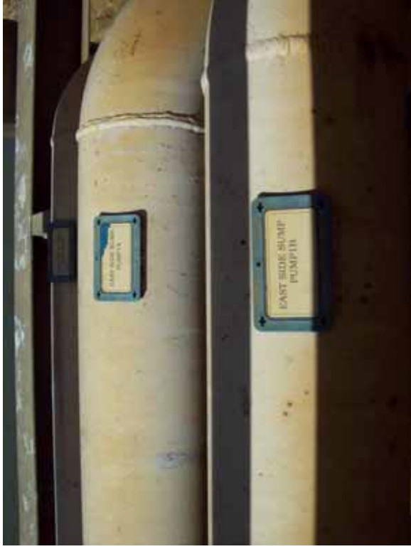
Photo 40: Labels for middle three 6-inch-diameter inlets shown in Photo 38.
