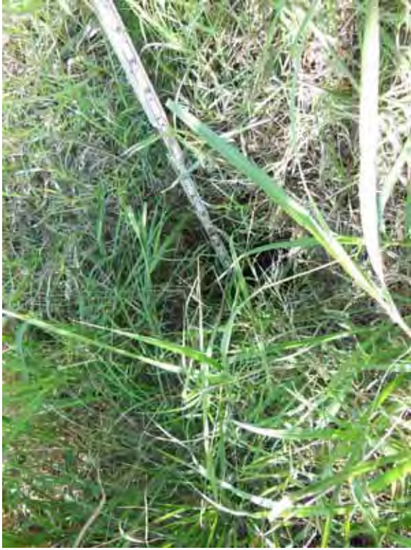
Photo 78: Approximately 18-inch-deep animal burrow at west embankment exterior slope.
