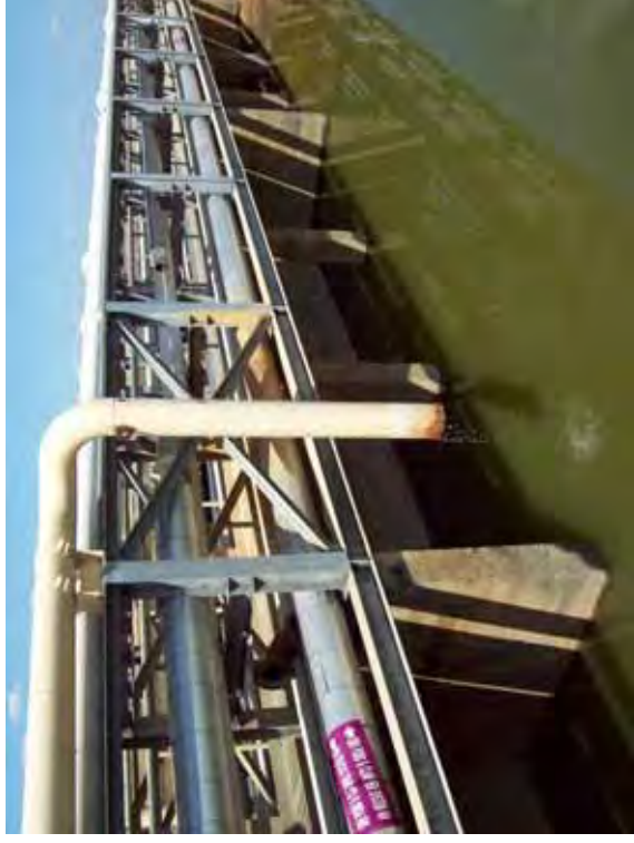
Photo 26: 8-inch-diameter metal SRH-south inlet pipe labeled "Plant Drain System III", looking northeast.
