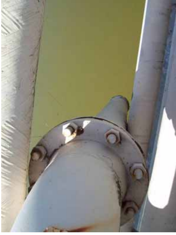
Photo 42: 6-inch-diameter metal SRH-north inlet pipe labeled "Waste Slurry Sump", looking north.
