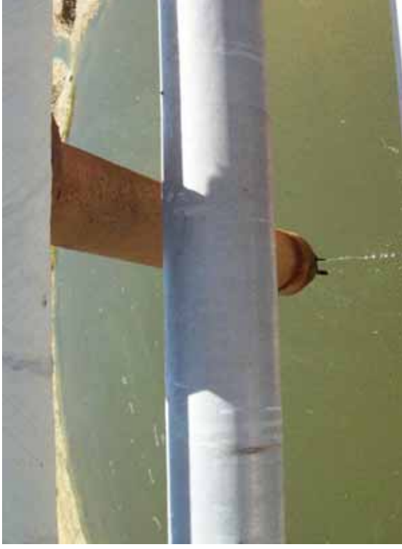
Photo 30: 6-inch-diameter metal SRH-south inlet pipe, looking south.
