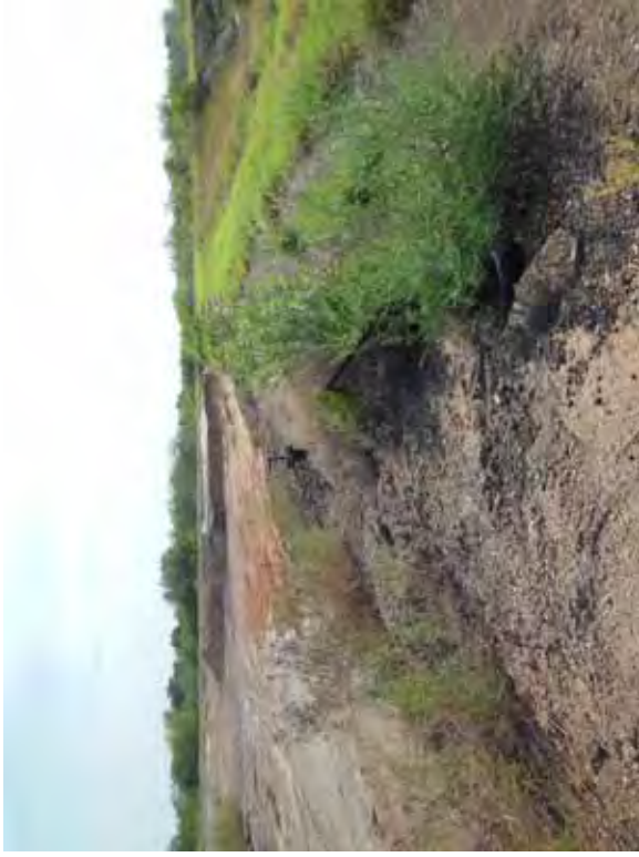
Photo 86: South embankment exterior slope measured approximately 3H:1V.
