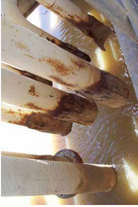
Photo 34: Nine outlet pipes into SRH-south, looking south.
