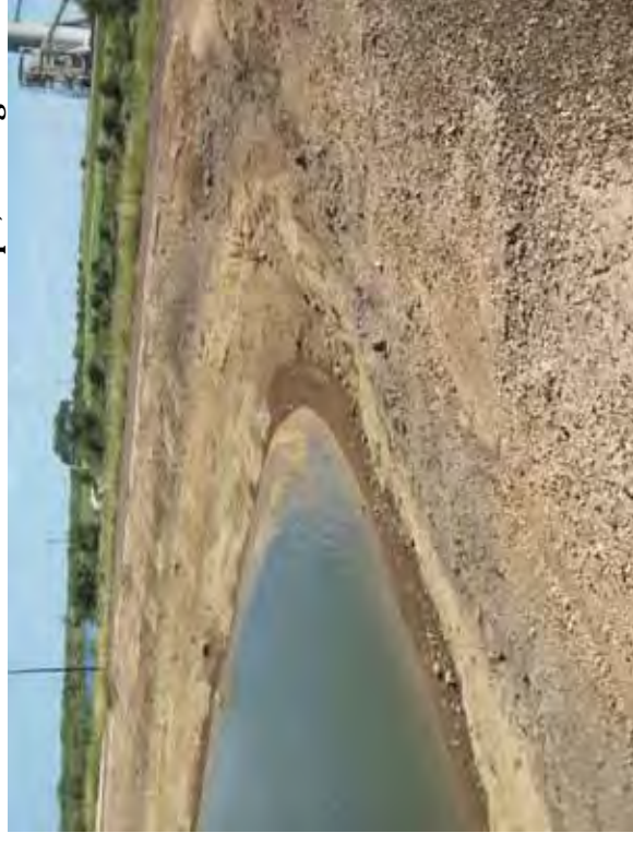
Photo 48: Interior slope at southwest corner interior slope, looking southeast.
